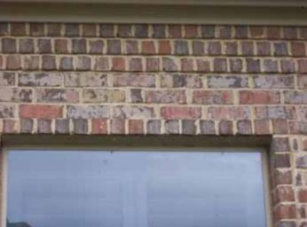
No weepholes over the garage door and window steel lintels.
