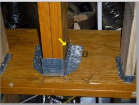
• One or more joist hanger(s) were observed to be missing over the media room wet bar area.
