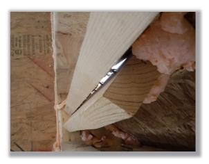
• The are doubled / tripled upped studs missing in the single car garage to line up below the load baring supports in the bedroom above it. It is recommended to ad additional stubs to help with transferring the load to the foundation.
