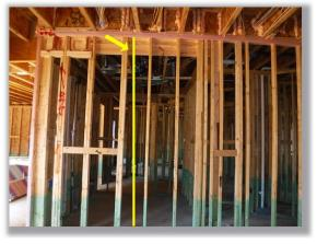
• The bathtub blockouts are missing / damaged at and around the tubs in the upstairs northeast bathroom and upstairs northwest bathroom.
