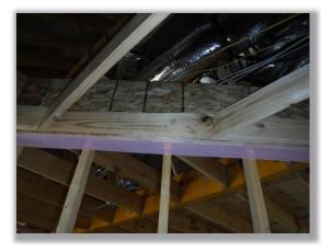
• The platform in front of the upstairs attic access needs to be better blocked to prevent someone from damaging ceiling finishes.
