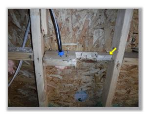
• The joist hanger over the gameroom is not properly fastened in place. There are larger gaps on both sides of the joist and the fasteners to not secure the joist.
