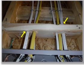
• The wires are not properly secured in place to hole the wires 1 1/2-inch from the edge of the stud face. The wires that need to be secured are located in the garage, family room and study.
