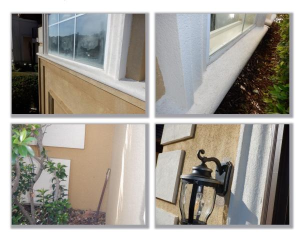
• The stucco has poor clearance from the concrete flatwork. Under current installation standards, there should be at least 1.5-to 2-inches of clearance between the concrete flatwork and the stucco material. There are no visible defects related to this application at this time and no remedial repairs are recommended.
